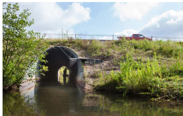
Figure 2.3.1.5: Wildlife shelf is installed in a culvert near Boonville, N.Y. Kurt Gardner/The Nature Conservancy via AP.
