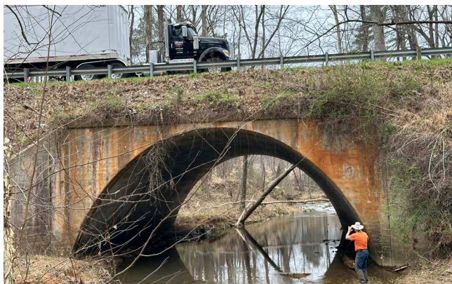
Figure 2.3.1.3: Bottomless culvert at US 70 over Stony Creek. DCHC MPO.
