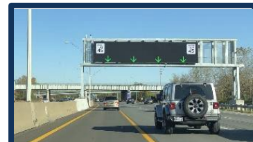
E. Hard Shoulder Running
