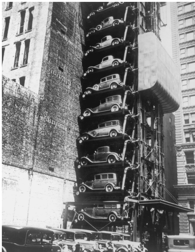
The “vertical parking machine” of 1932 could hold 48 cars. Hulton Archive, via Getty Images
