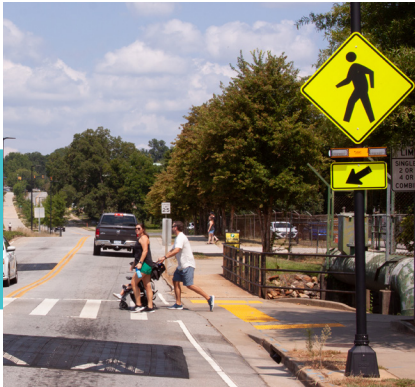
Rectangular Rapid Flashing Beacon (RRFB)
