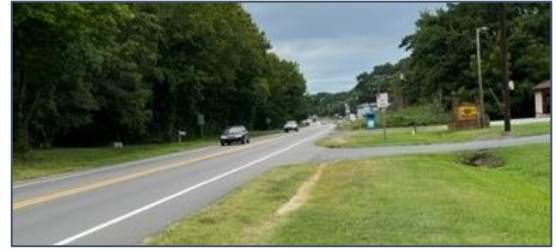
Worn path observed west of US 70 Business
