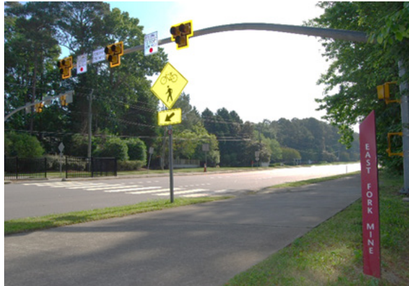
High Intensity Activated Crosswalk (HAWK)
