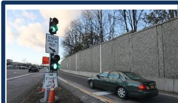
B. Ramp Metering
